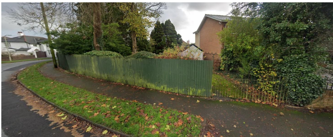
Fig. 2: Street View image of the application site
